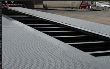
Floor Plate Decking with Open Frame Center
